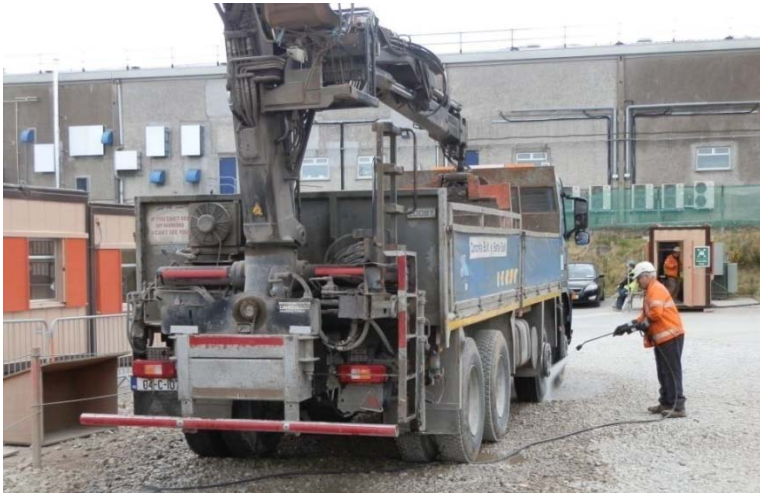
Figure 5.3 – Example of wheel washing of truck as it leave site
